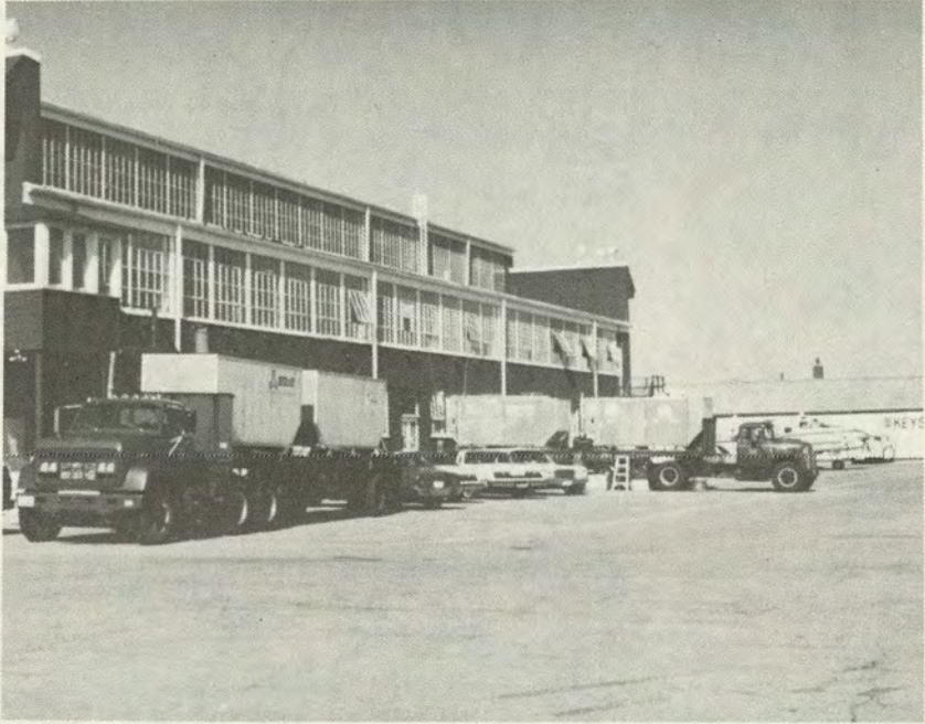
Pennsylvania Department of Transportation hangar at Capital City Airport. The large containers on the trucks contain communications and technical equipment.
